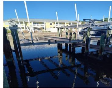
Boat Lift can accommodate 13,000 lbs and up to a 32 foot boat
